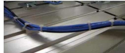
The only acceptable method for binding Cable / Wire / Optical Cables / Tubes is to use cable holders. Cables and tubes shall be tightened to the cable holder. The cable tie shall go through both sides of the holder. For single wire it is allowed to use just one side.
