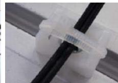
Distance between cable holders < = 120 mm Short connections between optical sensor and transmitter are also allowed. No coiling of the cables, if proper cut to length is possible. Exceptions can be announced in special cases.
